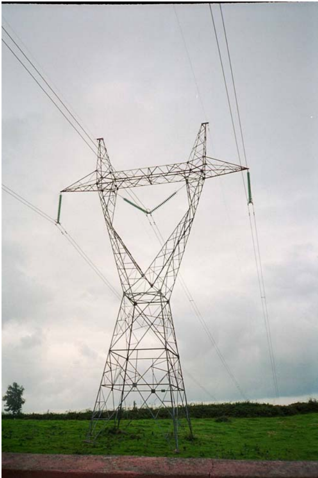
Indicative 400kV Single Circuit Intermediate Tower
