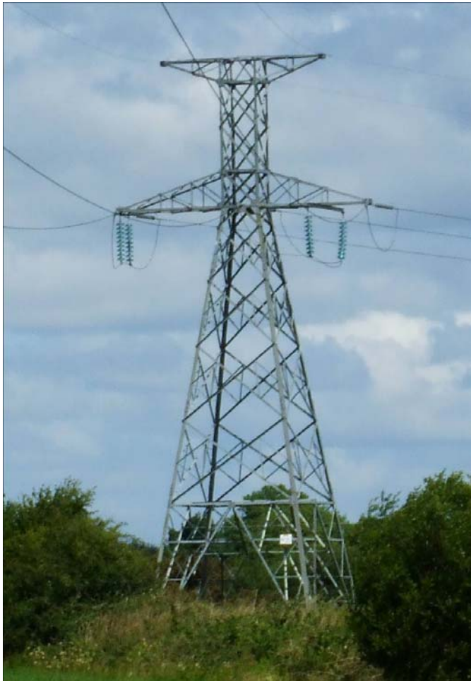
Indicative 110kV Single Circuit Angle Tower
